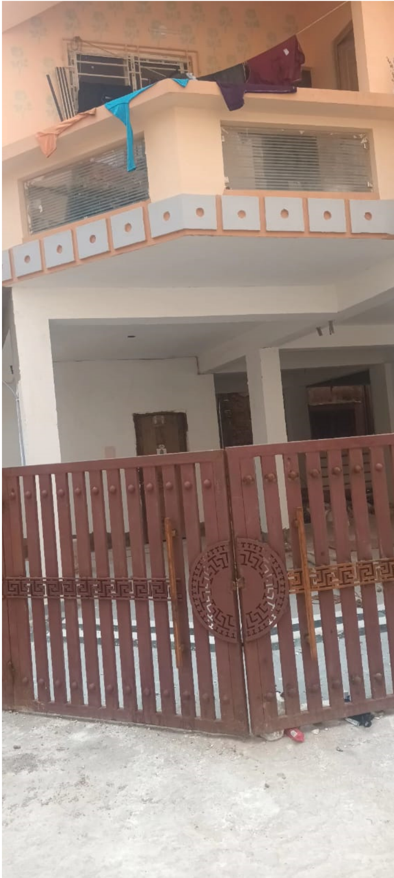
ASHA RESIDENCY_GROUND FLOOR & PASSAGE WORK_COMPLETED
