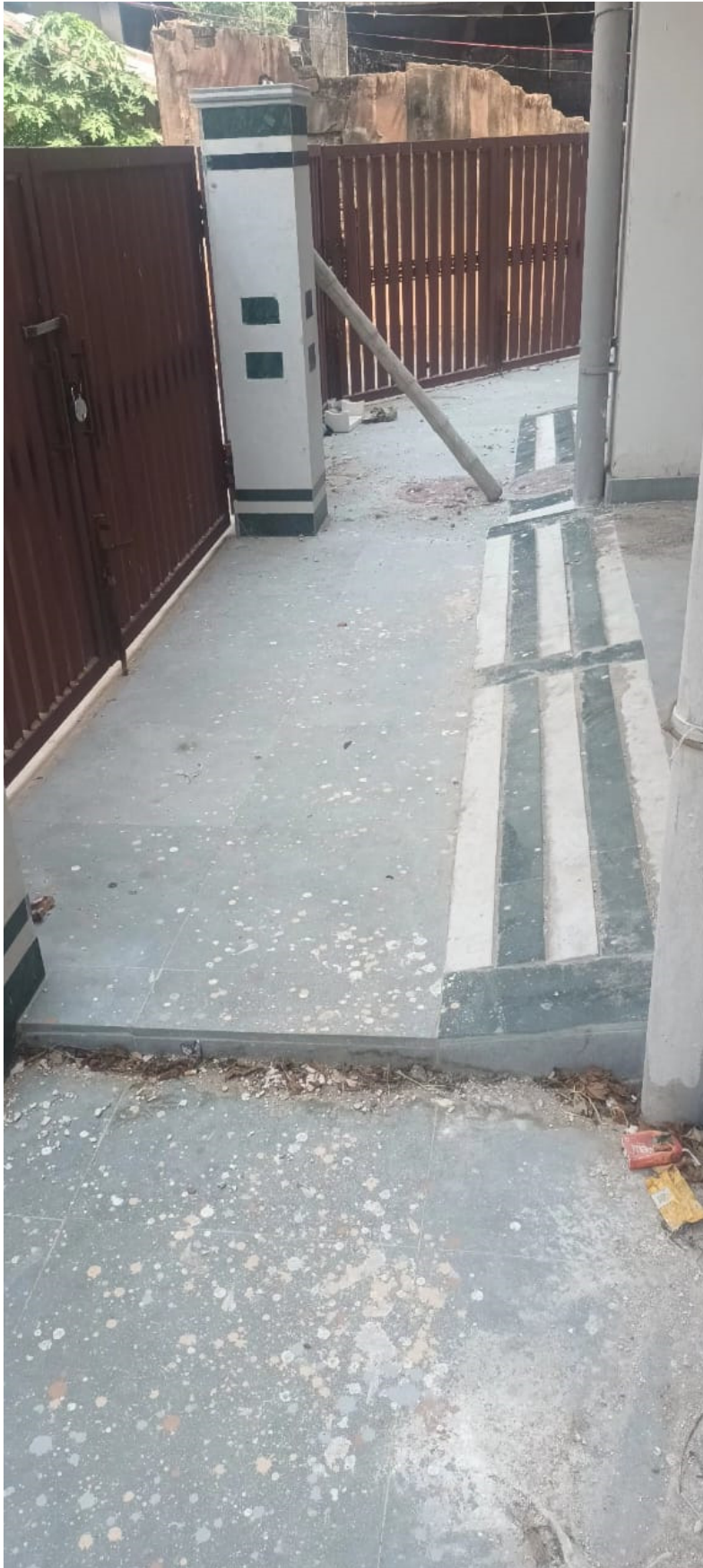
ASHA RESIDENCY_GROUND FLOOR & PASSAGE WORK_COMPLETED
