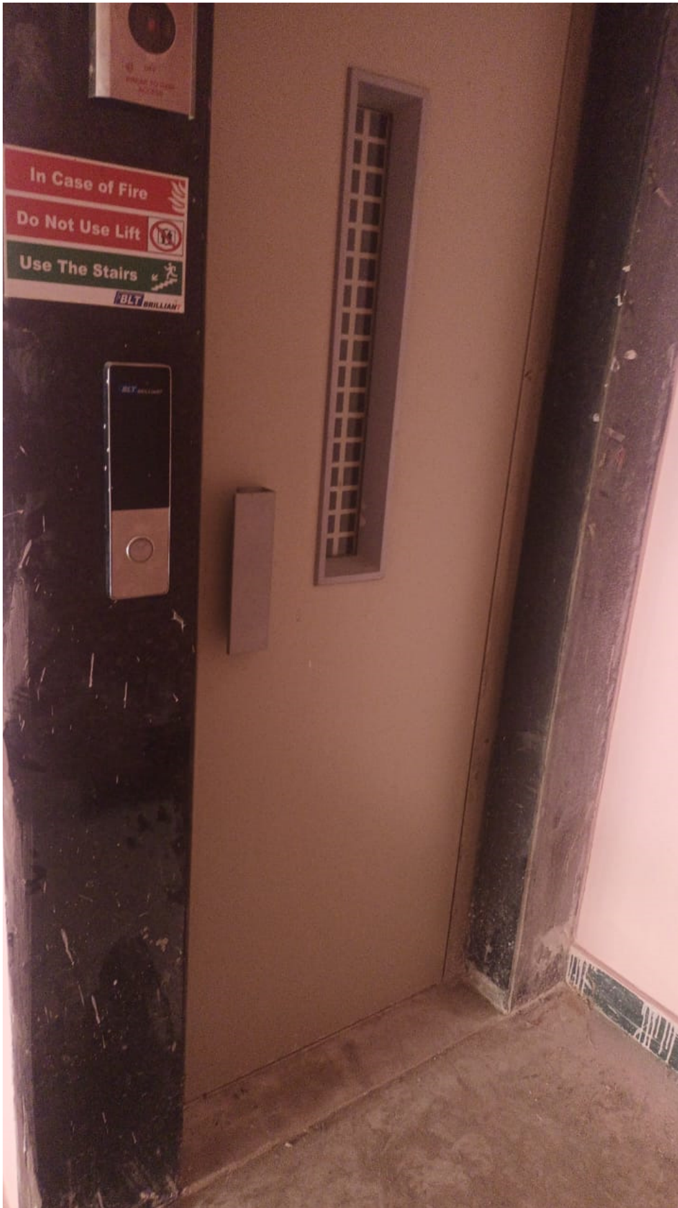
ASHA RESIDENCY_GROUND FLOOR & PASSAGE WORK_COMPLETED
