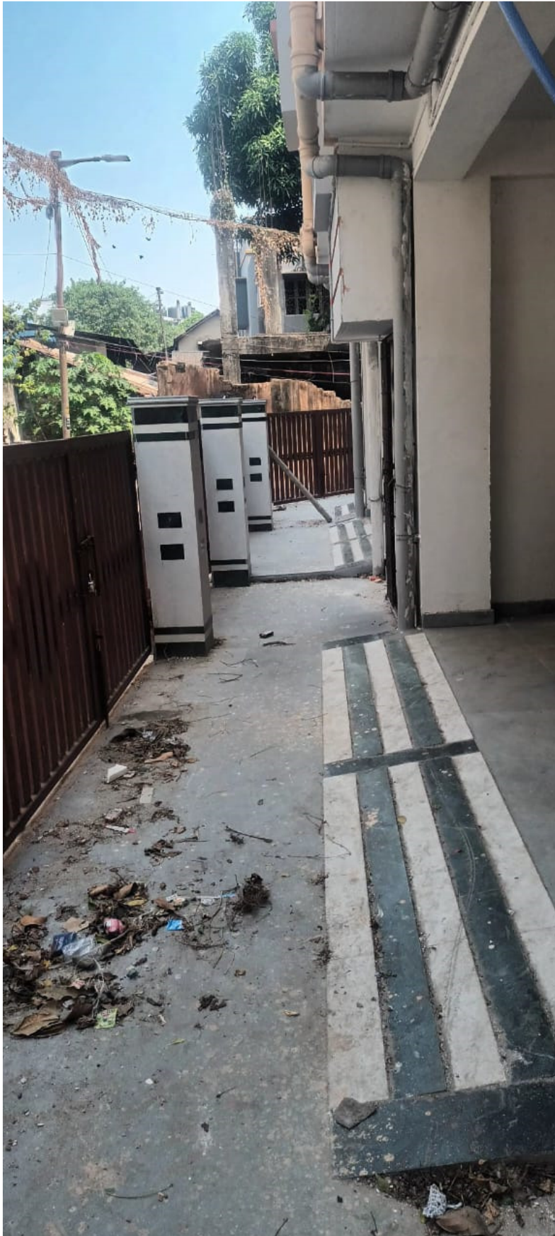
ASHA RESIDENCY_GROUND FLOOR & PASSAGE WORK_COMPLETED
