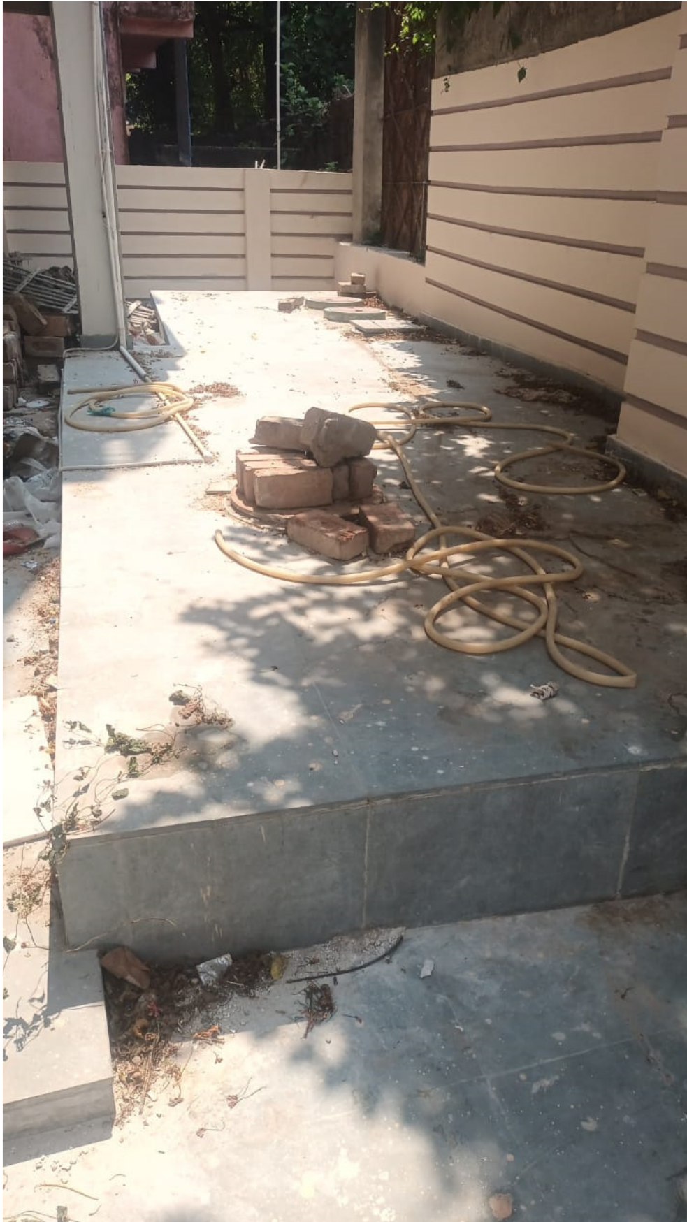
ASHA RESIDENCY_GROUND FLOOR & PASSAGE WORK_COMPLETED
